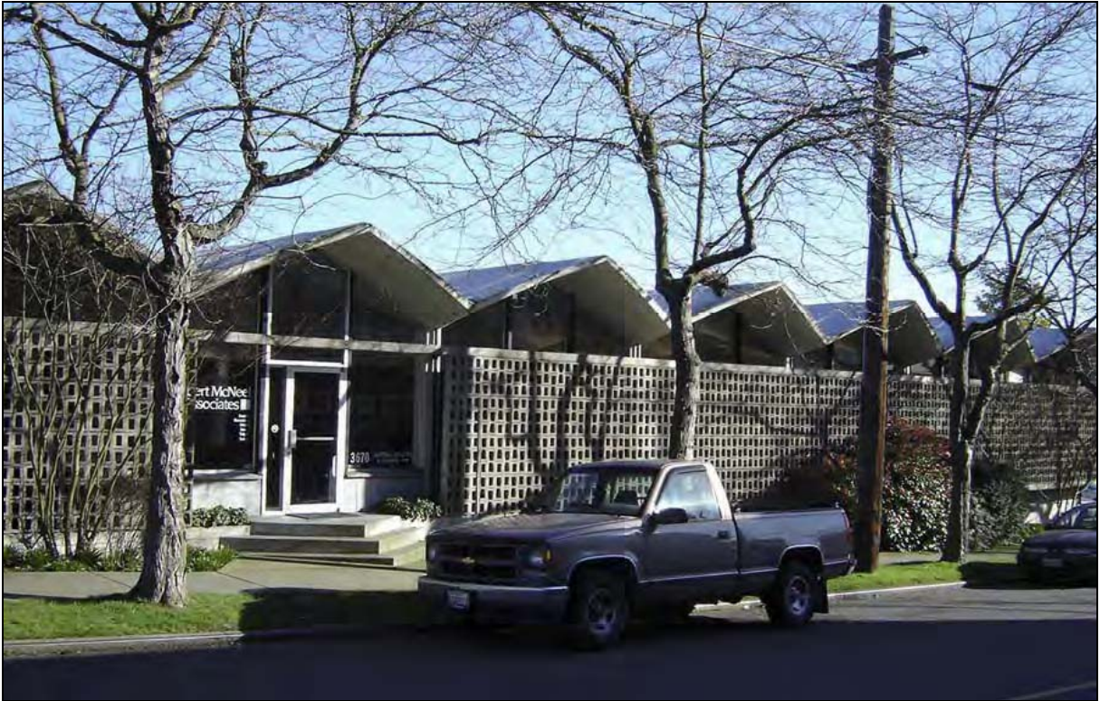
Figure 37. Above, a view looking southeast at a portion of the west facade in January 2006.
