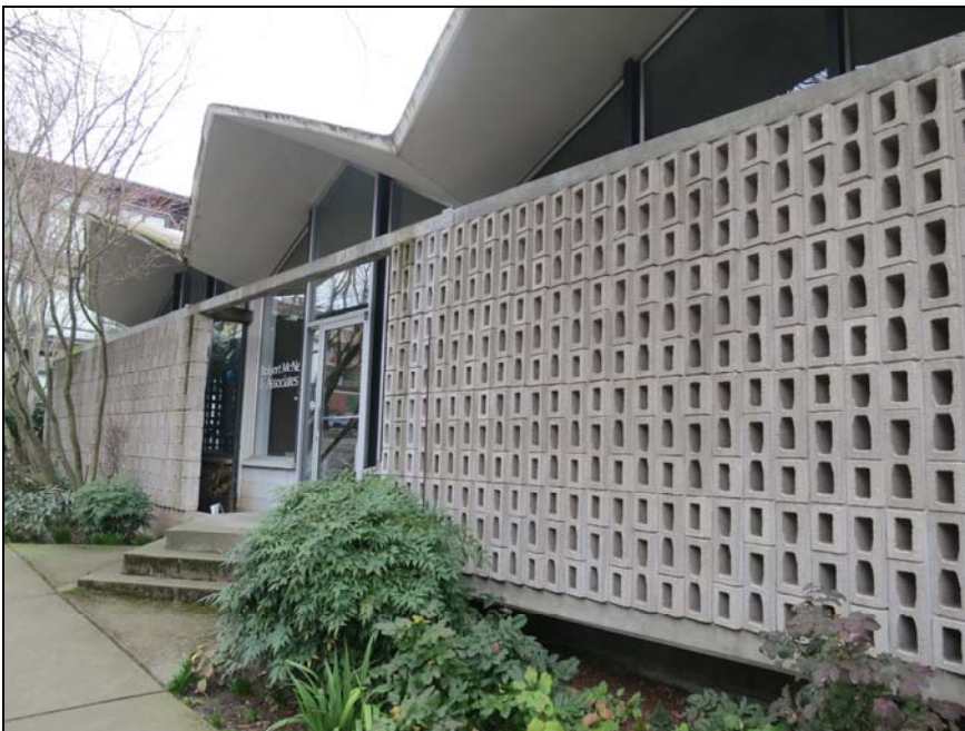
Figure 38. Below, a detail view along the west facade at the west entry.
