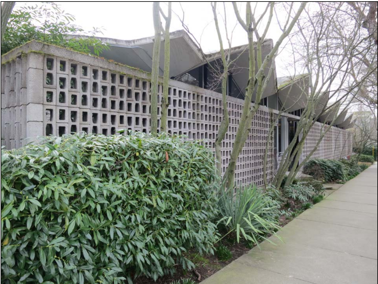
Figure 41. Below, an oblique view looking southeast at the northwest corner and west facade.
