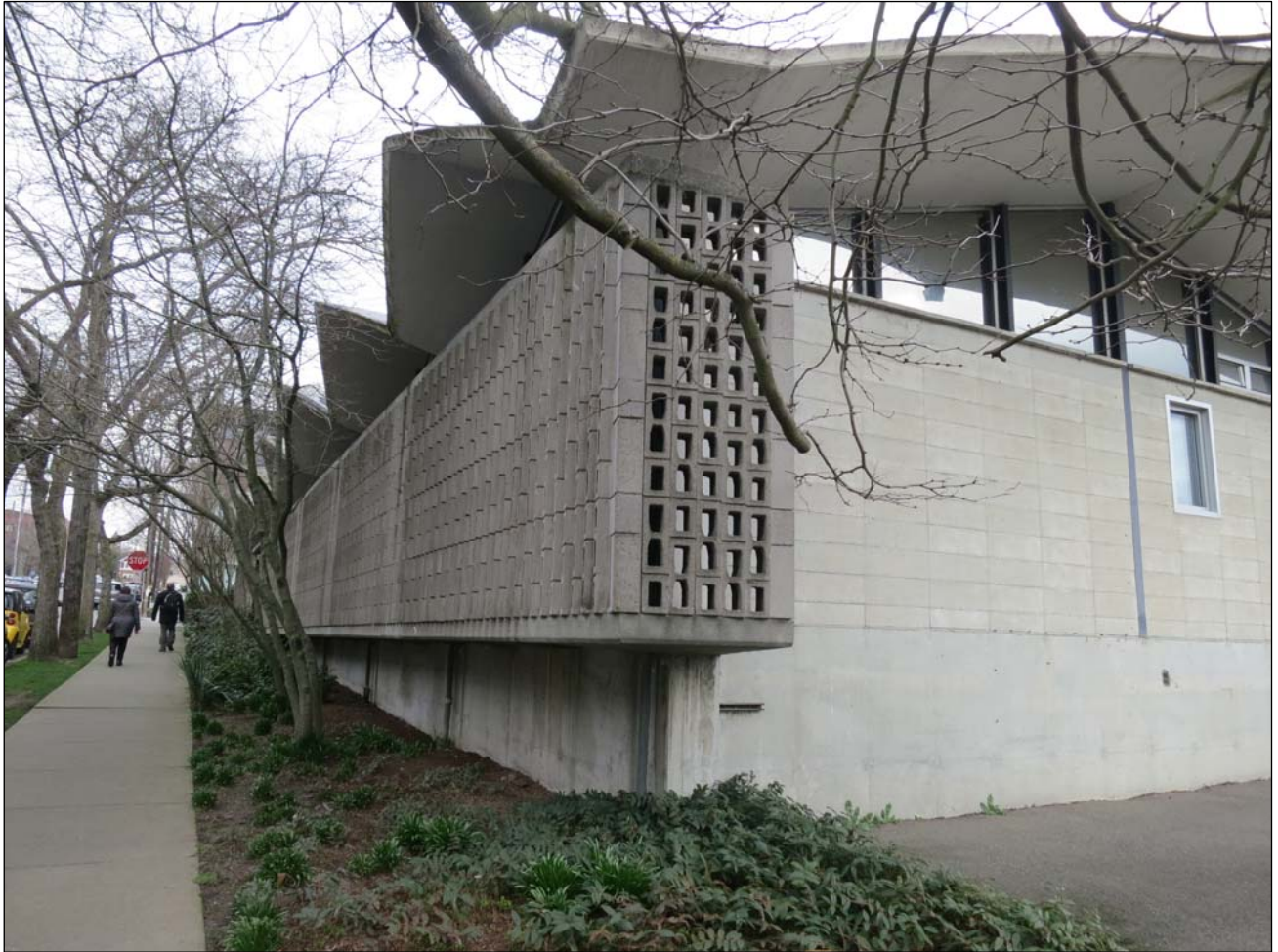
Figure 39. Above, a view looking north at the building's southwest corner, showing portions of the west and south facades, projections of the folded plate roof structure, and the cantilevered slab and screen wall, which turns this corner, and plant beds along the sidewalk of Woodland Park North.
