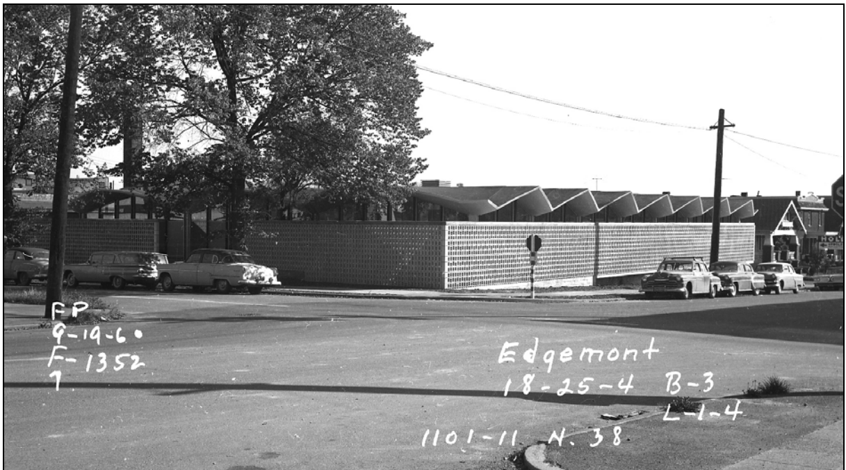
Figure 29. Below, the King County Tax Assessor's Property Record Card photograph of September 19, 1960 (Puget Sound Regional Archives).
