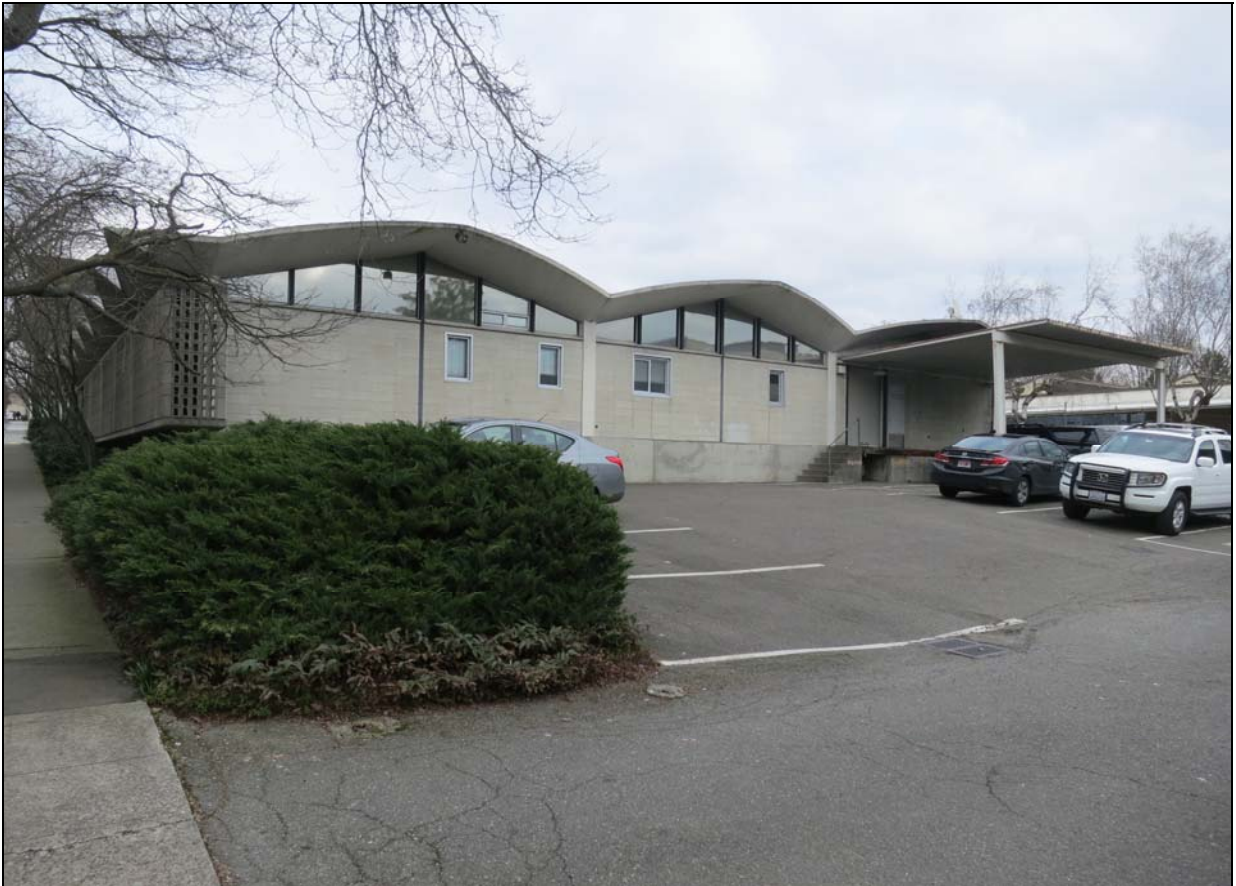
Figure 44. Above, looking north at the south facade and adjacent parking lot. Clerestory windows are original, while smaller windows in openings in the stacked block wall represent recent additions.
