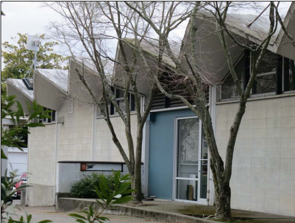
Figure 43. Below, a detail view of the non-original east entry, also shown in the photo above.
