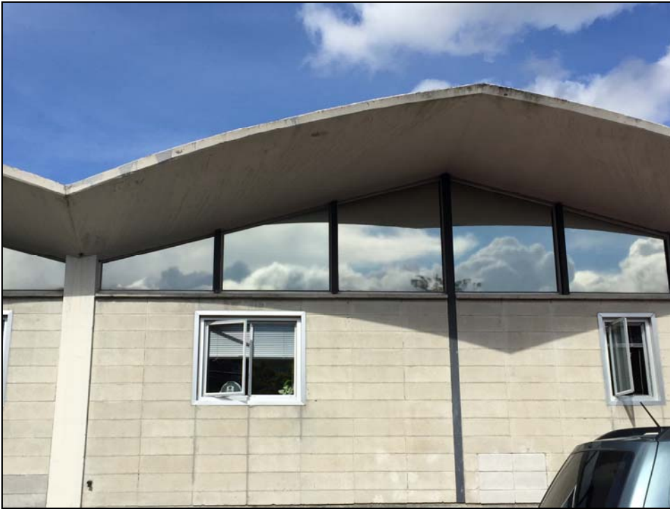
Figure 48. Detail view, south façade, showing the clerestories below projecting roof and non-original windows in mid- 2015.
