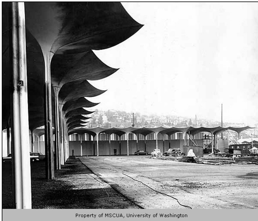
Figure 15. Below, temporary thin shell canopies under construction for the Century 21 World's Fair in 1961 (UWLSC).
