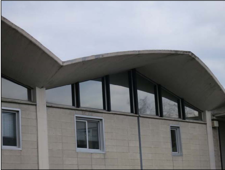
Figure 53. Above, a detail view of the south façade, roof edge and clerestory window.
