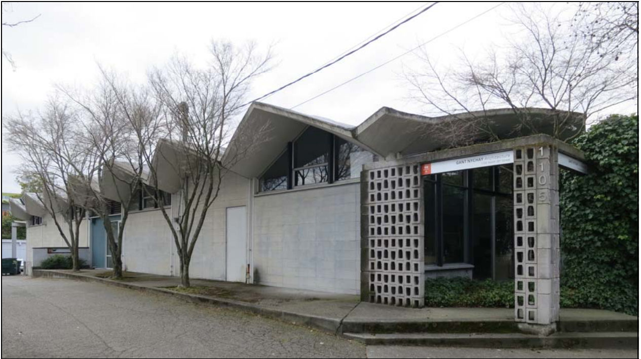
Figure 42. Above, an oblique view looking south at the east facade.
