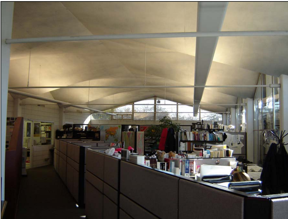
Figure 54. Below, interior view looking south toward the clerestory windows in office in 2005.
