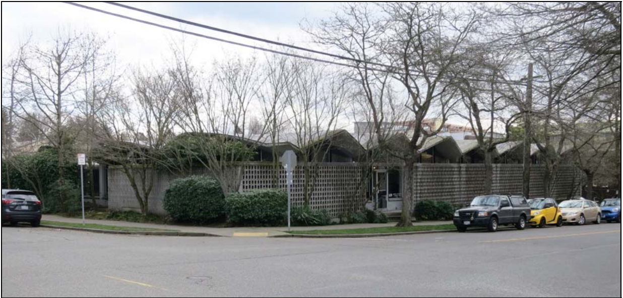
Figure 40. Above, view looking southeast at the property and the west and partial north facade.
