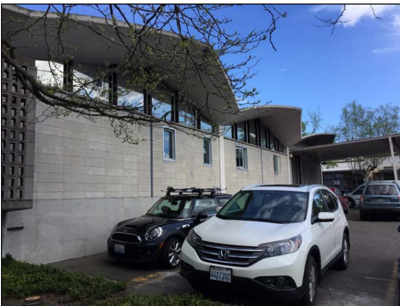
Figure 45. Below, oblique view looking northeast at a portion of the south facade in 2015.
